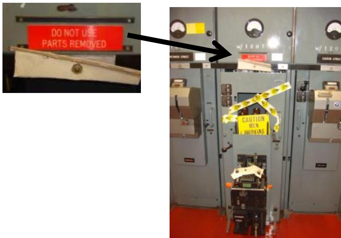
Photograph 10 – Example of parts having been removed from an obsolete 11kV circuit-breaker at SSEPD’s Lochee primary substation
