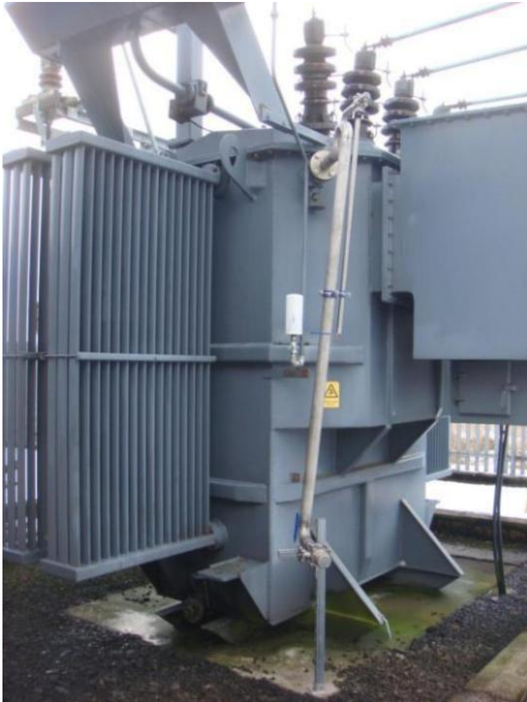
Photograph 3 – Temporary pipework at SSEPD's Leoch primary substation
