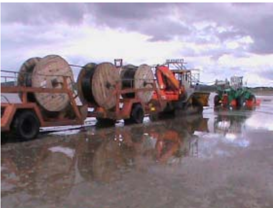
Figure 7 Cable plough in operation in Islay
